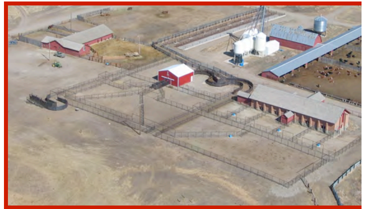
Figure 1. Aerial view of Northern Agricultural Research Center's entire cattle handling facility, constructed in summer 2007. Cattle handling capacity is 400 pairs.
