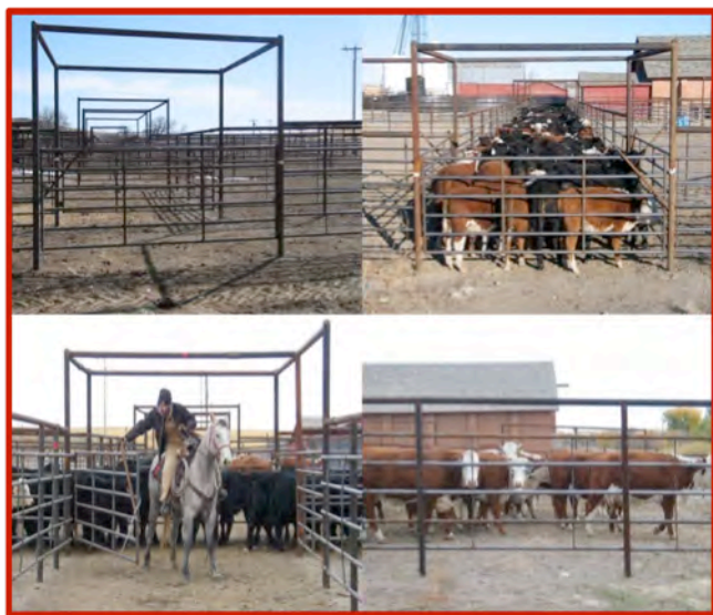
Figure 3. Pipe overheads and posts with 6-rail continuous fence.
