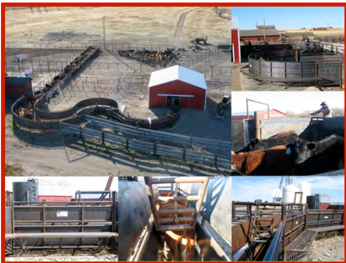
Figure 2. Curved alley, crowding tub and single file race with adjustable backstops and catwalk on the inside of the curve.
